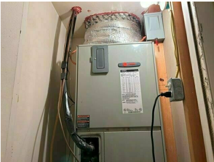
53. View of typical HVAC and water heater closet in three bedroom apartment
