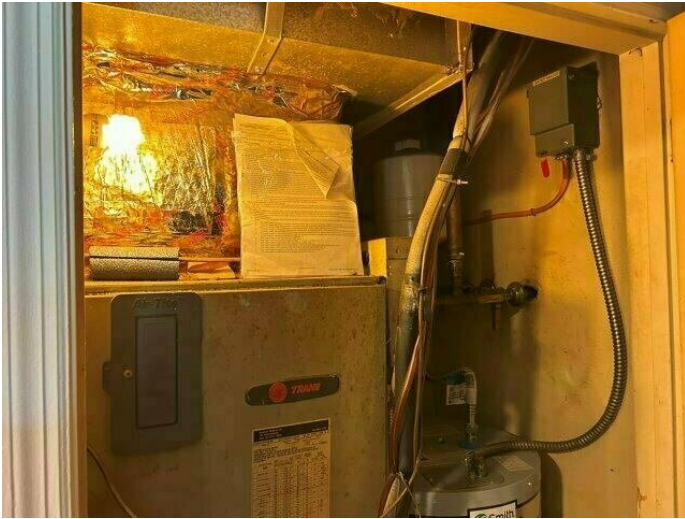
49. View of typical HVAC and water heater closet in one and two bedroom apartments
