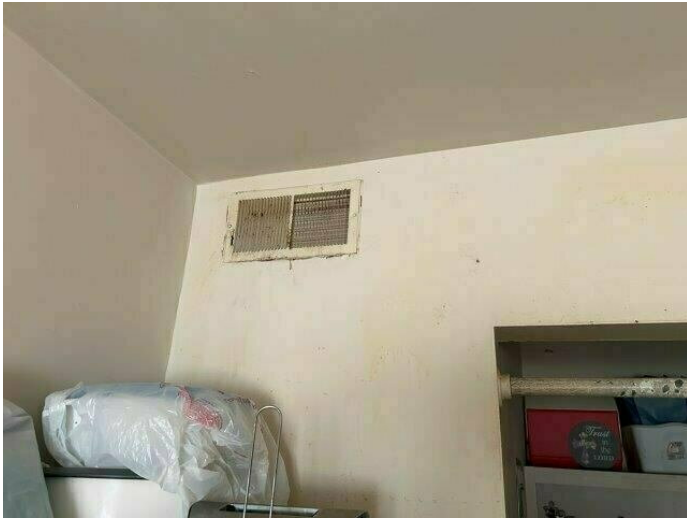
31. View of microbial growth and water damage
